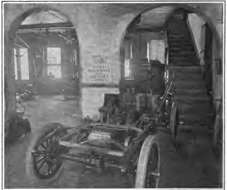
CORNER OF J. A. PLACE'S REPAIR SHOP IN GENEVA—TRANSFORMED CAR IN FOREGROUND.
